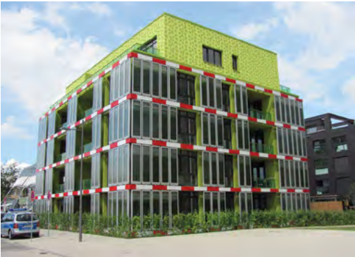
fig. 47 BIQ's bioreactor facade powered by algae.
