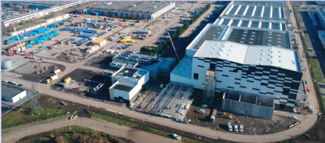
La gigafactory (ACC) en construction. Source : CABBALR
