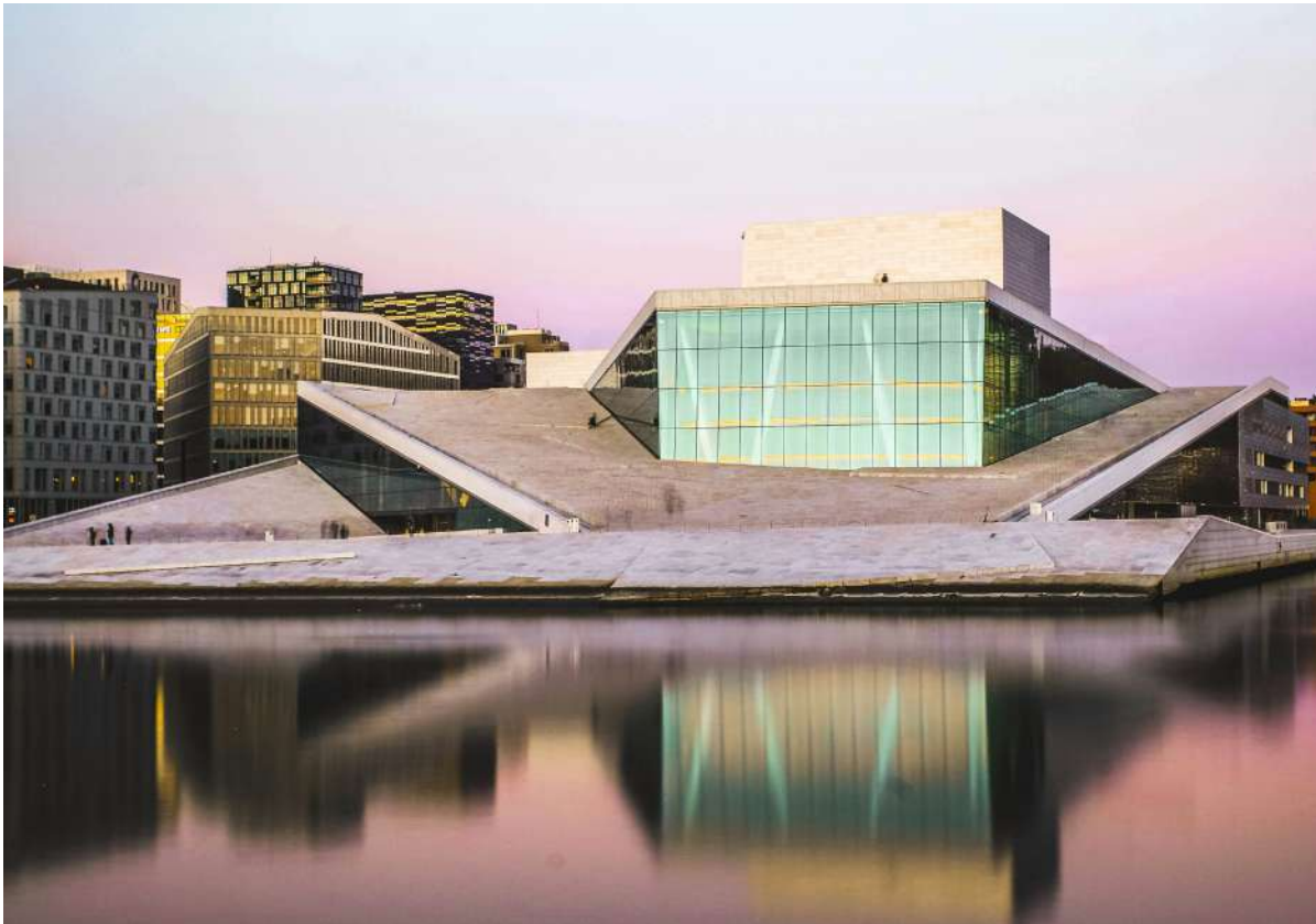
→ The Oslo Opera House
