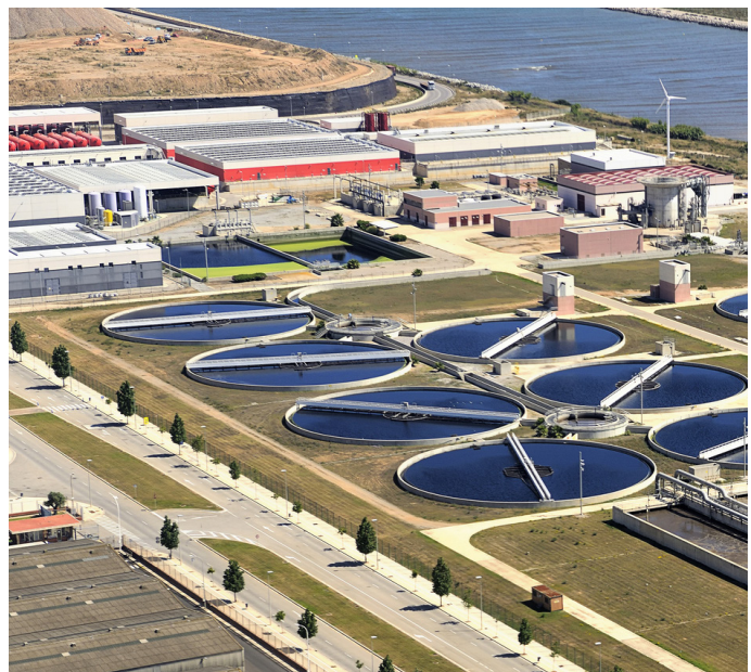
→ Llobregat Desalination and Regeneration Plant
